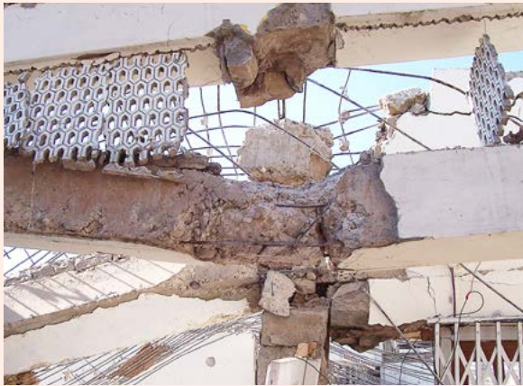
Damaged reinforced concrete building, impossible to repair and complex to retrieve salvage materials. Source: GOAL.
