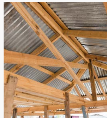
Strengthening roofs in Caribbean to avoid recurring damage in hurricanes. Source: CRS.
