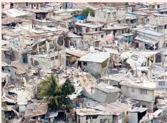
Entire neighbourhood destroyed in 2010 earthquake, Port au Prince, Haiti. Source: UN-Habitat.
