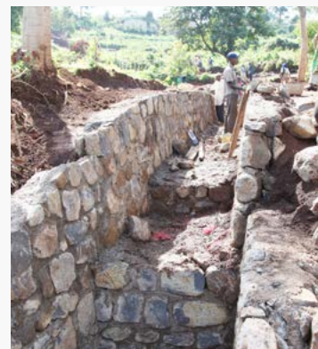
Settlement drainage and infrastructure works mitigate flooding. Source: UN-Habitat.
