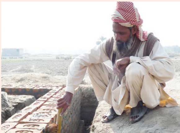
Mason pointing fired brick foundations for house reconstruction on raised platform in an effort to mitigate flood damage to the new house. The area has been affected by severe floods three times in ten years. Source: UN-Habitat.
