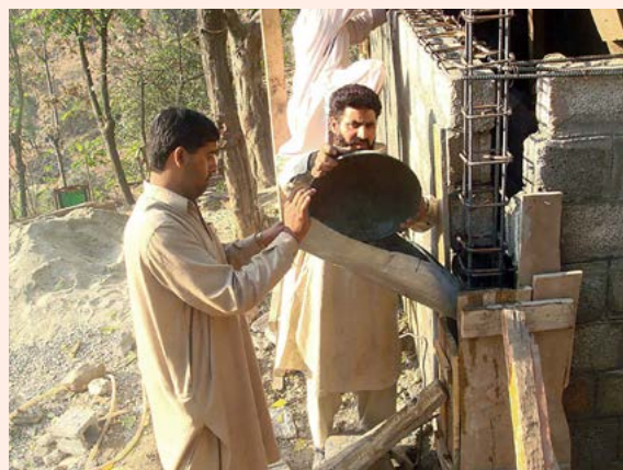
Engineer and mason in joint practical training. Source: UN-Habitat.
