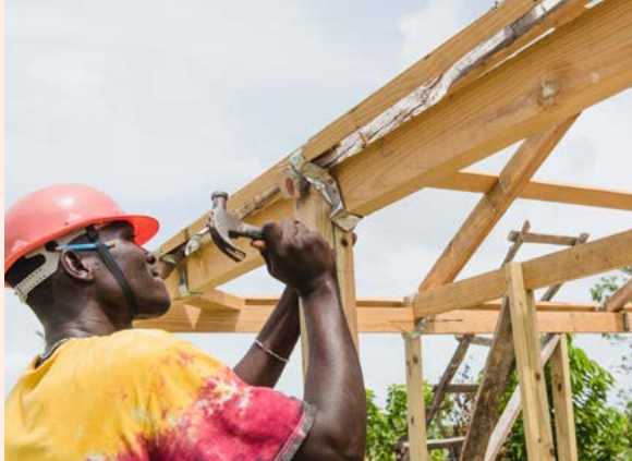
Carpenter installs hurricane straps. Source: CRS.
