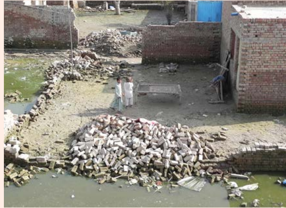
Flood recovery involved rehabilitation of boundary walls and improved area planning and drainage. Source: UN-Habitat.
