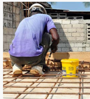
Steel fixer on demonstration house roof. Source: J/P HRO.
