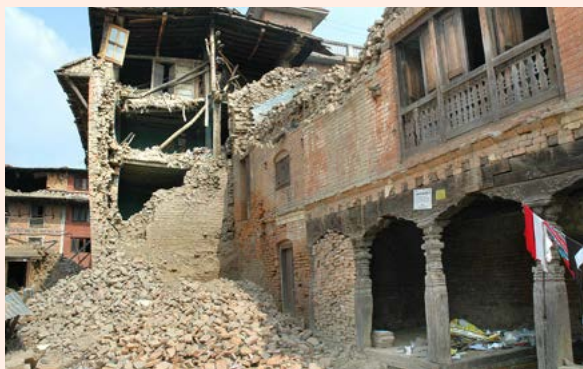
Houses, workshops, and community buildings damaged by the 2015 earthquake in the historic town of Bungamati, Nepal. 2015. Source: Shelter Cluster Nepal.
