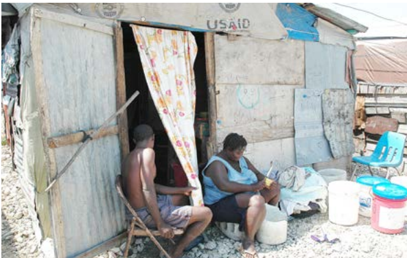
Shelter constructed by household using plastic sheeting and salvaged materials. Source: Shelter Cluster Haiti.
