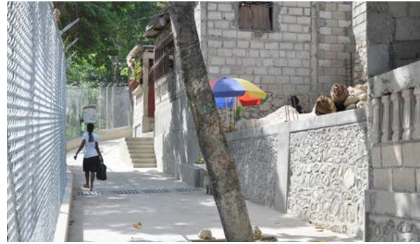
Ravine in informal neighbourhood of Campeche after investment in improvement measures to improve circulation and drainage, and to reduce solid waste disposal and flooding risk. Upgrading infrastructure in residential neighbourhoods supported housing and settlement recovery. Source: UCL.
