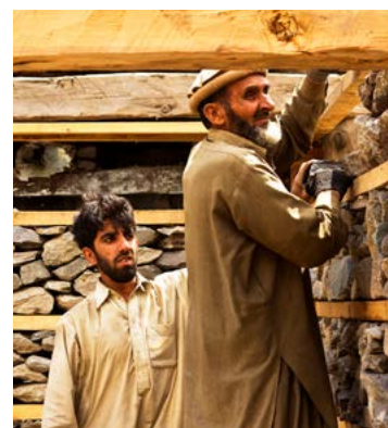
Reviving traditional knowledge of earthquake resistant techniques in local materials. Source: UN-Habitat.
