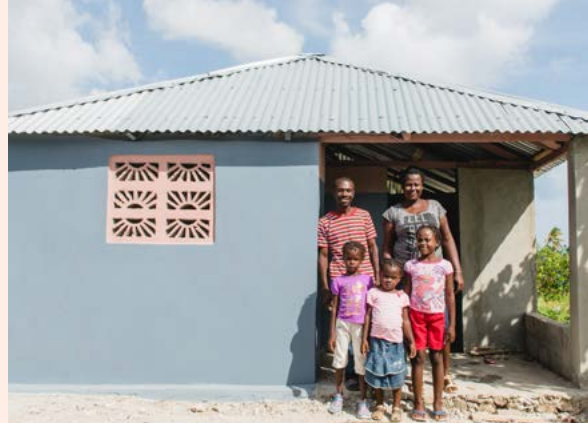
Fully reconstructed new house. Source: CRS.
