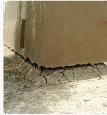
Low strength mud masonry. Difficult to develop standards to achieve resistance to flood or earthquake hazards. Heavy mud masonry buildings perform well on thermal and cost criteria. Source: UN-Habitat.
