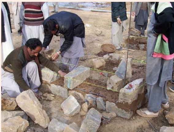
Training masons in traditional earthquake resistant stone masonry techniques. Pakistan. Source: GOAL Ireland.
