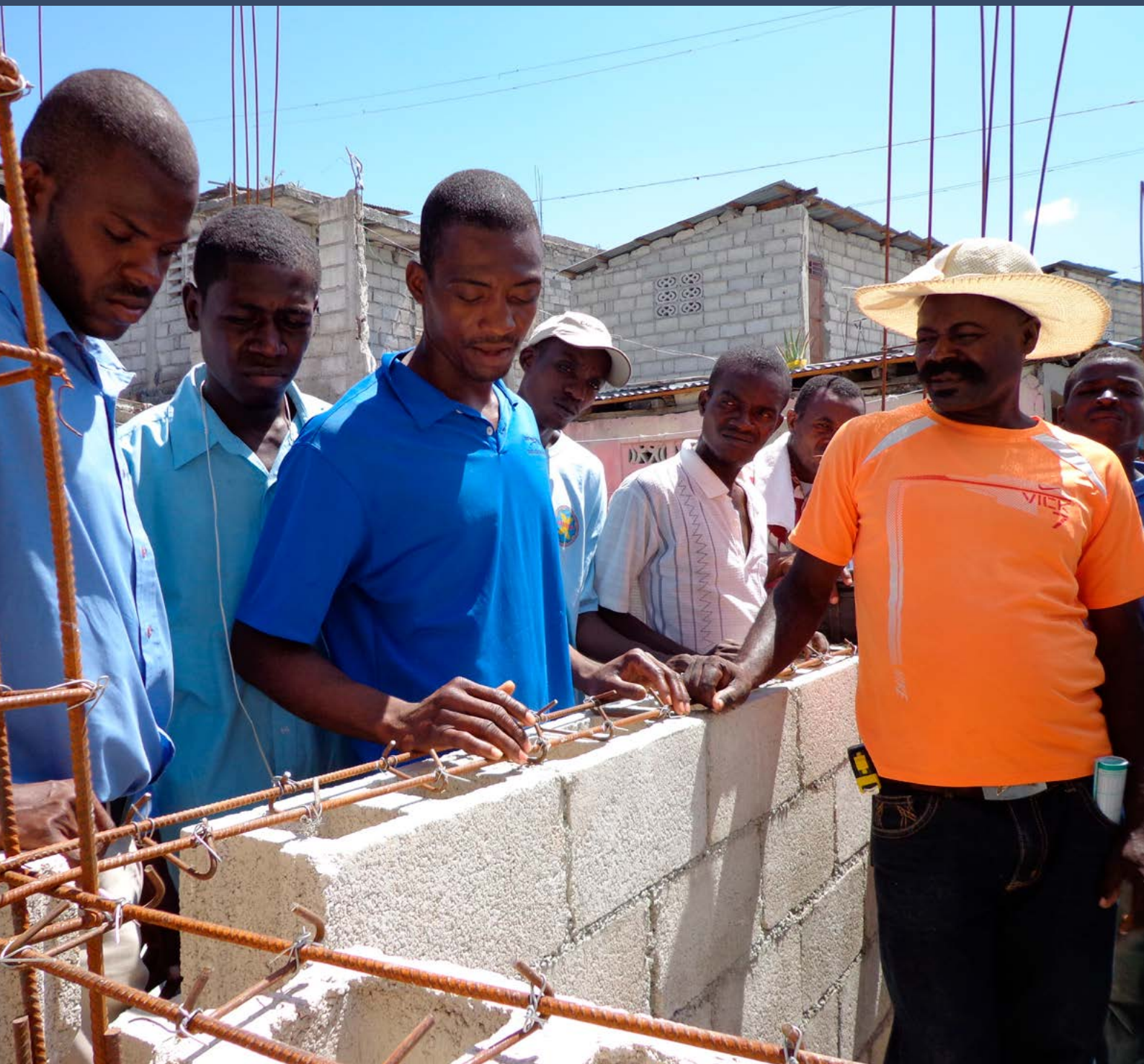
Visit to demonstration house and information event to learn safer construction standards and practical application.
