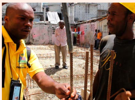
Government engineer on site in Delmas 32 explaining steel size information to local masons. Haiti. Source: J/P HRO.
