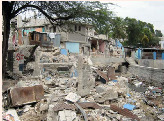
Damage in the neighbourhood of Ravine Pintade after the 2010 earthquake in Port-au-Prince. Source: Global Communities.
