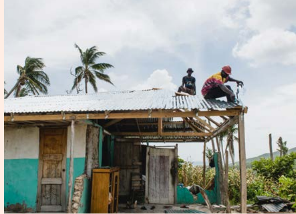
A mobile technical assistance team carries out repairs and strengthening on a damaged verandah roof. Source: CRS.
