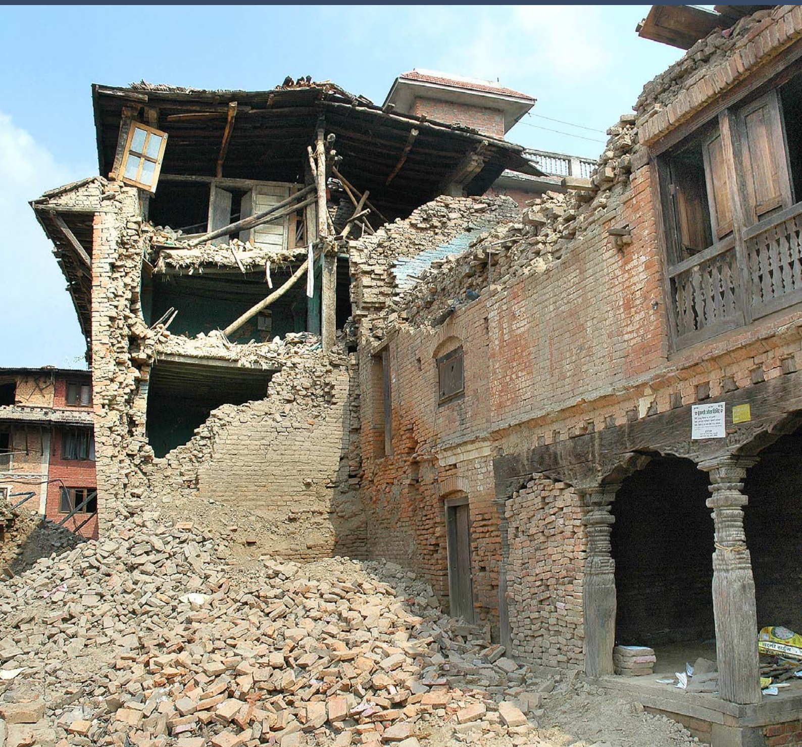
Houses, workshops, and community buildings damaged by the 2015 earthquake in the historic town of Bungamati, Nepal. 2015.
