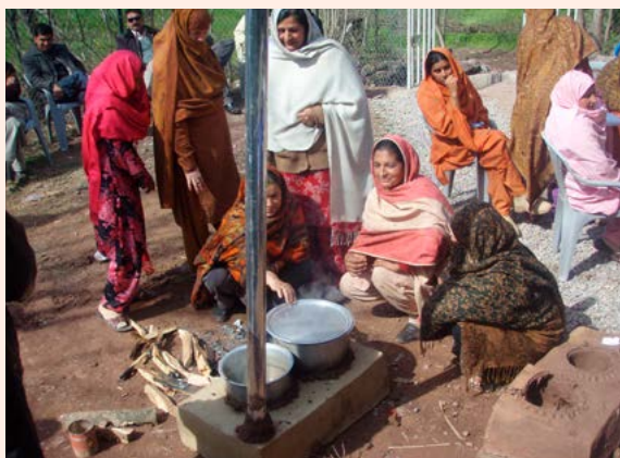
Women training women to build fuel-efficient stoves during housing reconstruction after the 2005 Kashmir earthquake. Pakistan. Source: UN-Habitat.
