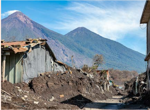
Clearing access for the road and to property after slides. Guatemala. Source: CRS.
