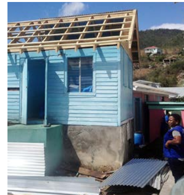
Rebuilding local timber framed house after Hurricane Maria, Dominica.
