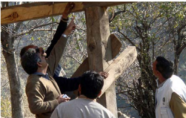
Senior government structural engineer investigating traditional timber construction details and performance of buildings during preparation of standards for reconstruction. Source: ERRA.
