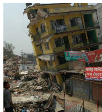
Urbanization increases the importance of compliance with regulations. Source: Shelter Cluster Nepal.
