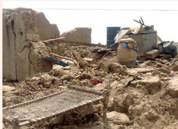
Standing water damage to adobe and mud masonry buildings. Source: UN-Habitat.
