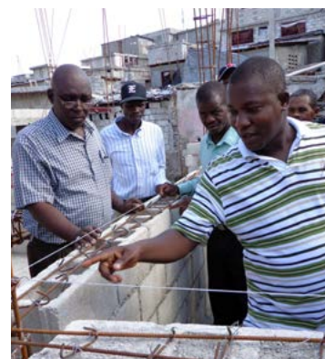
Government engineer on site at weekend event demonstrating standards for steel reinforcement.
