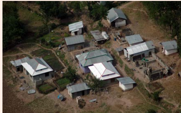
Houses reconstructed after 2005 Kashmir earthquake. Pakistan. Source: UN-Habitat.
