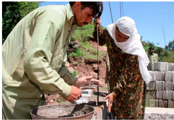
Woman checking the quality of mason's work on site, supervising construction of her own home. Source: Vero Wijaya/UN-Habitat.
