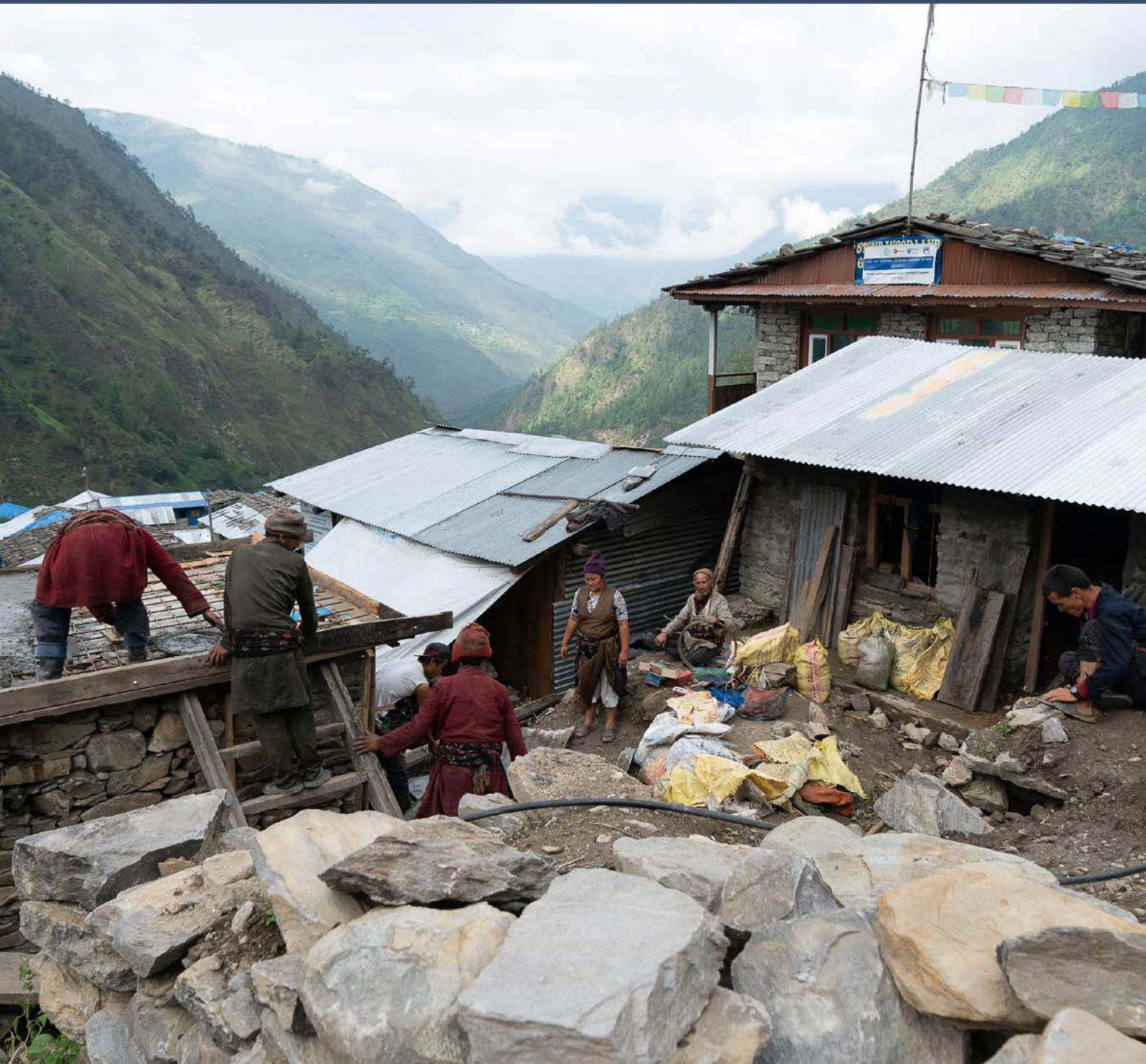
New houses reconstructed in accordance with building standards for stone masonry and interpretation of financial assistance conditions that households build individual houses. Source: Viv Cumming.
