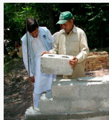
On-site advice to masons.
